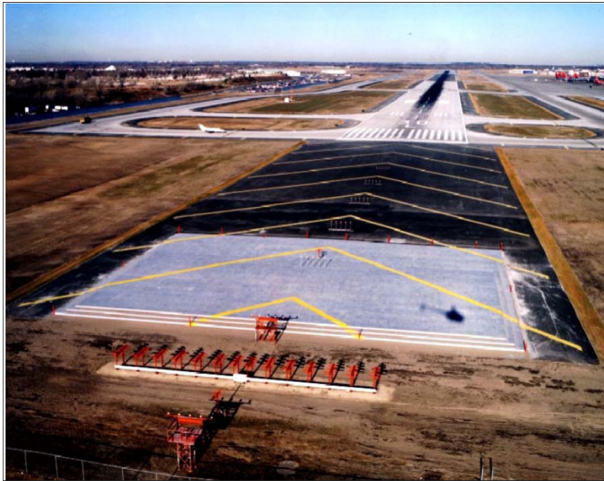
FIG 2-3-42 Engineered Materials Arresting System (EMAS)
